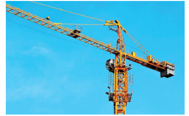
• 塔杆倾斜监测 Tower tilt monitoring
